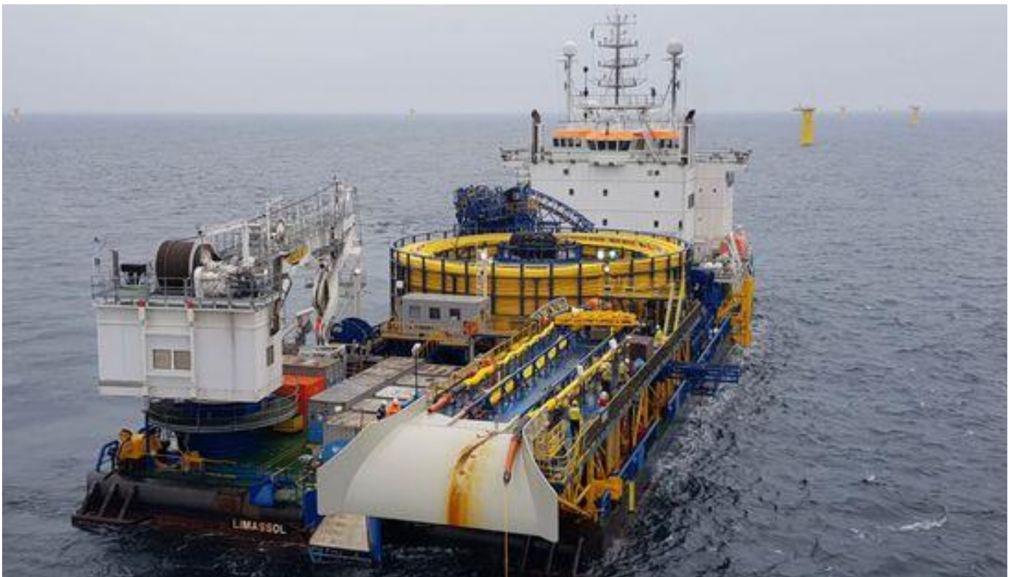
Figure 3.14: Example of inter-array cable installation at the EnBW Hohe See Offshore Wind Farm construction site in the German North Sea.
