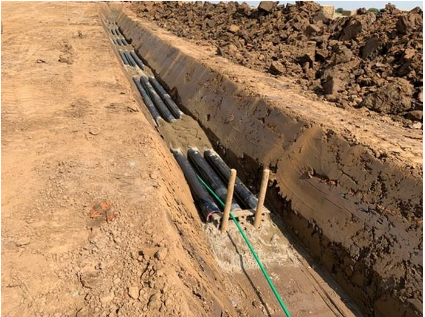
Figure 3.18: Example of an onshore export cable trench.
